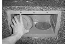
Turn Filter Counter-clockwise to Remove
