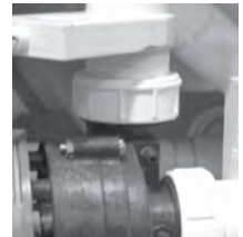
Slice Valve and Pump Union
