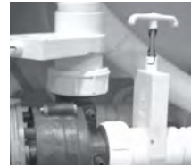
Slice Valve and Pump Union
