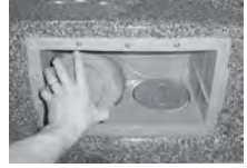
Turn Filter Counter-clockwise to Remove
